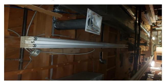
Photo 10 – Lower-level fluorescent lighting ballasts.
