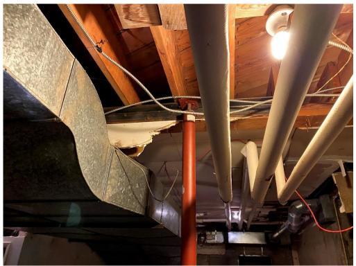
Photo 5- Support Post Below Old Bearing Wall Location
