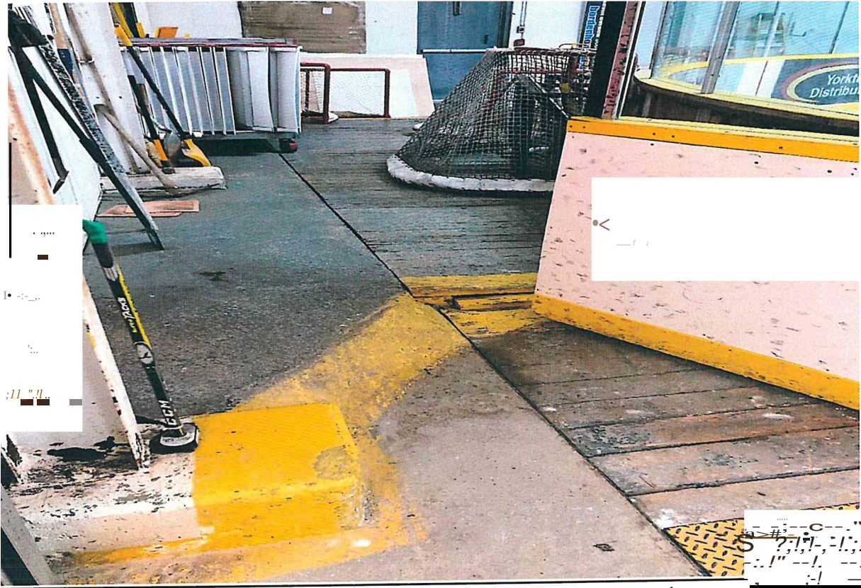
Picture #5 - Elevation variance on either side of ice resurfacer apron crossing.
