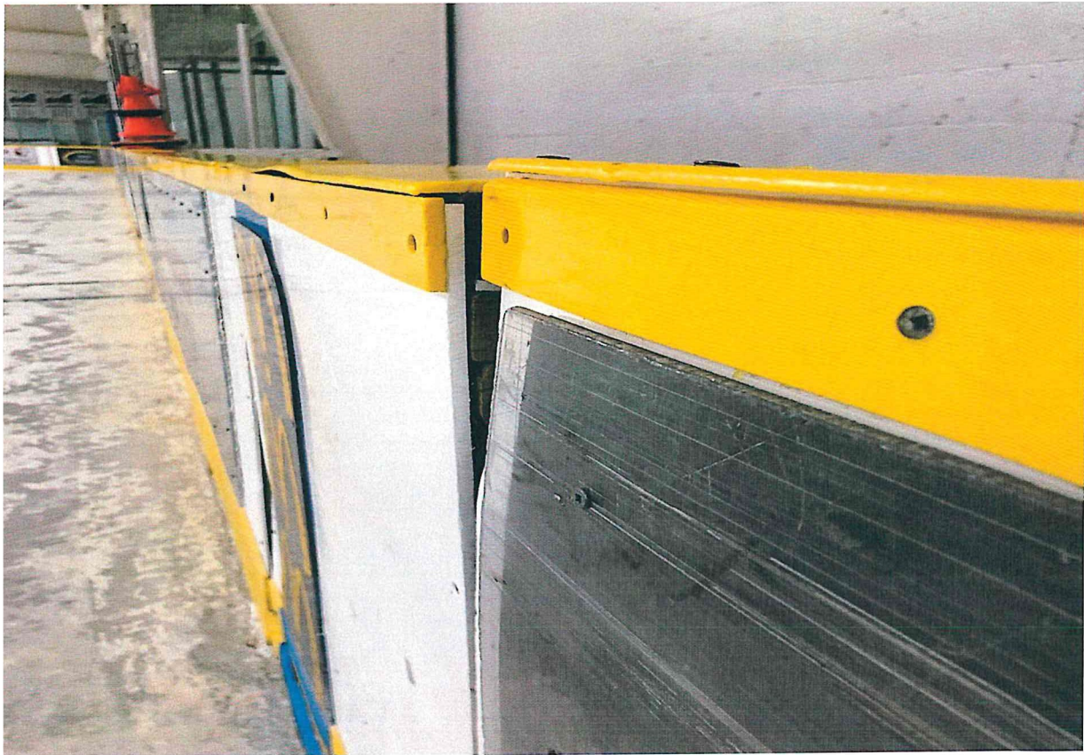
Picture #9 - On the north side the dasher board gates are not in line with the rest of the system and must be constantly adjusted to minimize risk to players.
