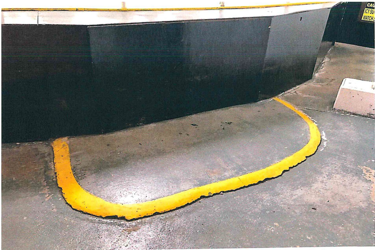
Picture #6 - Concrete topping represents a trip hazard.
