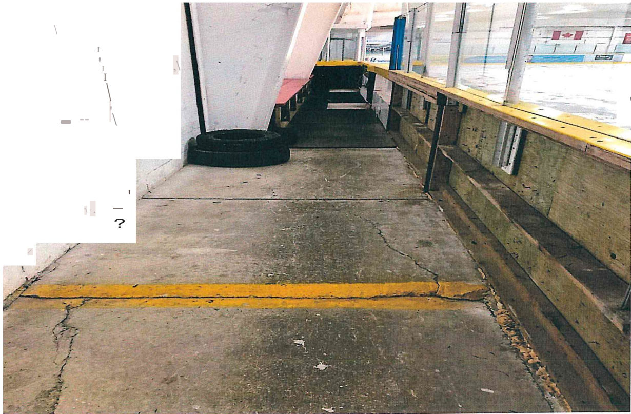
Picture #3 - Cracked walkway on north side.
