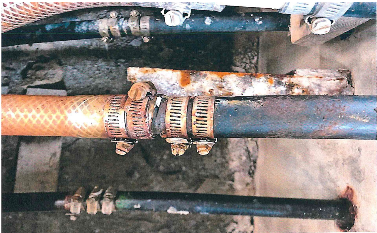
Picture #2 - Heavily rusted hose clamps are indicative of leaks and will fail over time.
