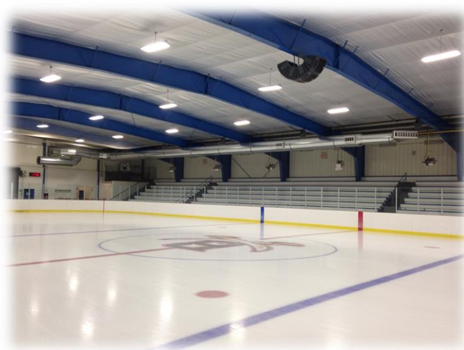
Dehumidifier Ductwork Inside Rink
