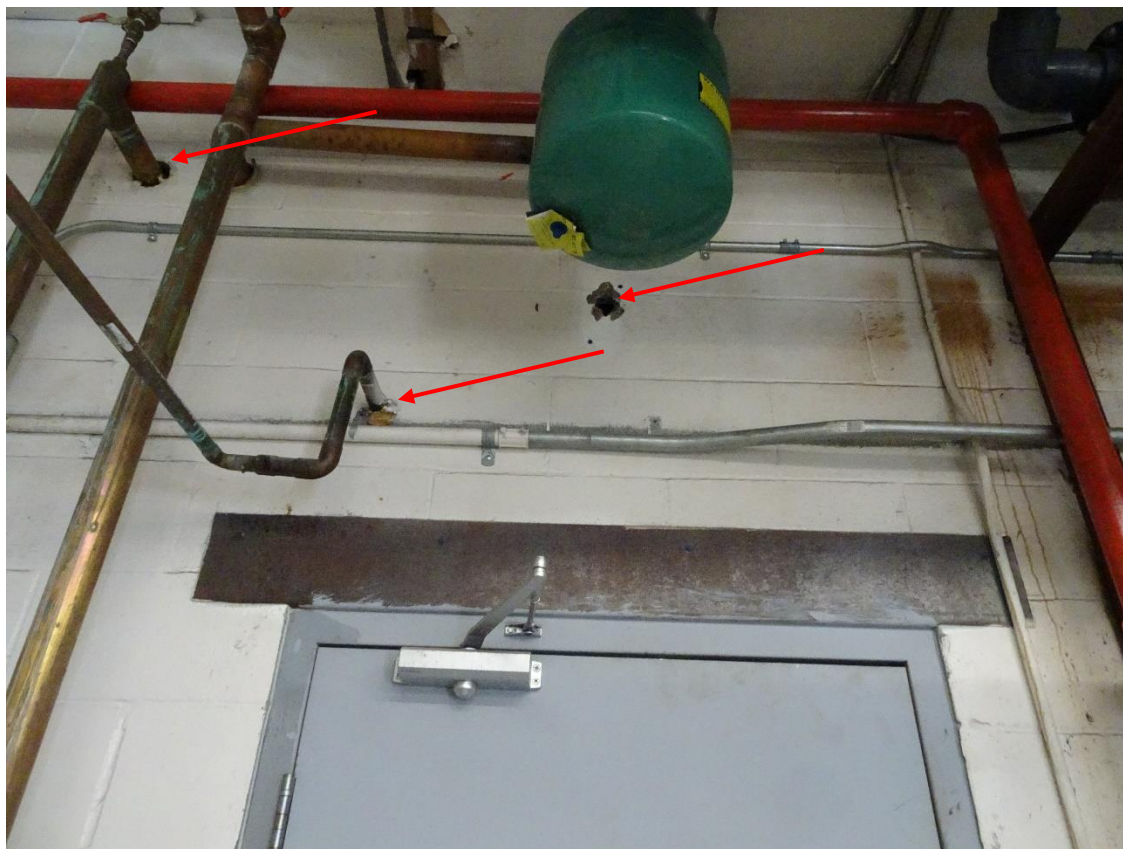
Figure 3 – Example of holes in walls
