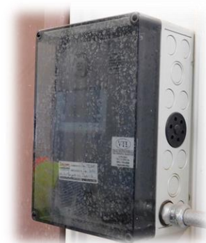
Zamboni Room Carbon Dioxide Sensor Unit
