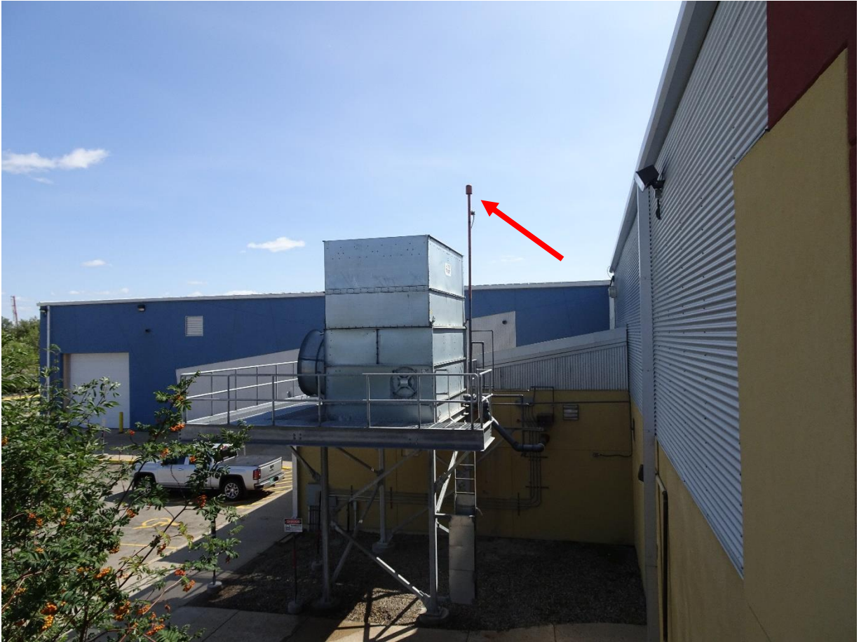
Figure 1 – Relief stack discharges towards ground.
