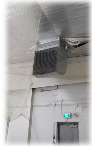
One of the Rink Exhaust Fan Openings Exhaust Fan is on Roof Above
