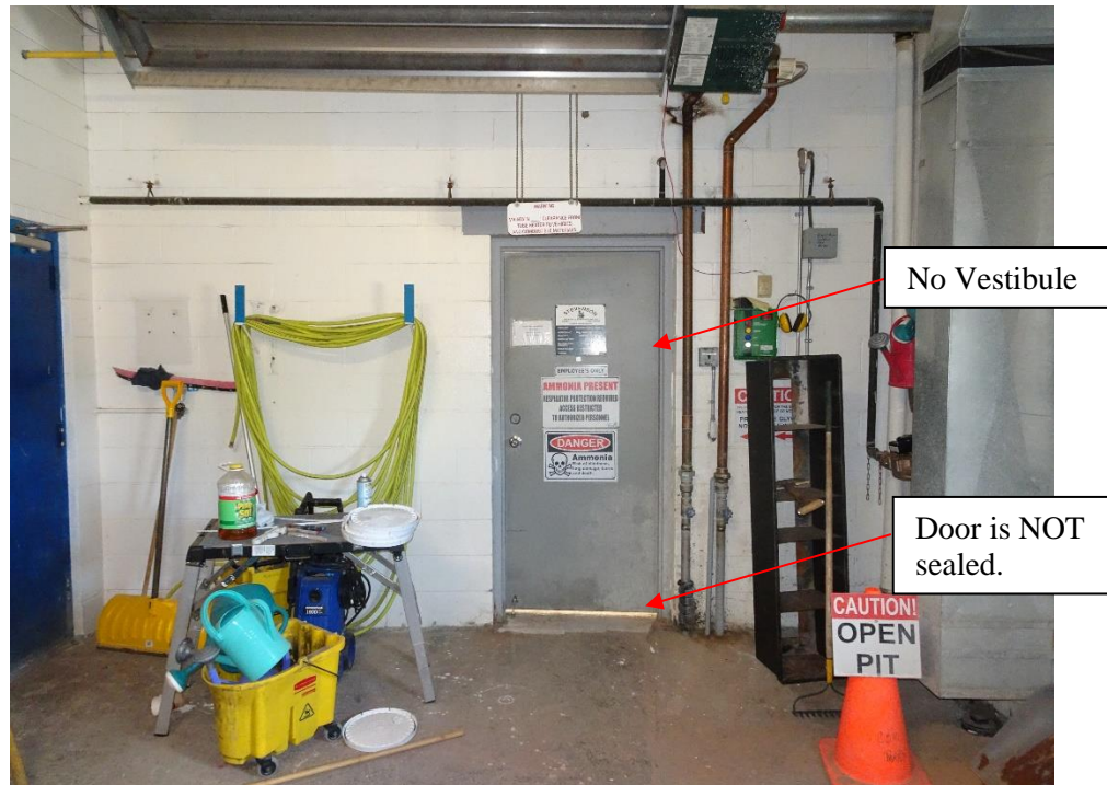
Figure 5 – Machine room door without vestibule.
