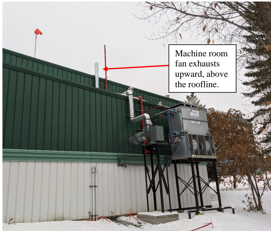
Figure 4 – Example of Ammonia Rink Ventilation system designed by SRCI to discharge above the building's roof.
