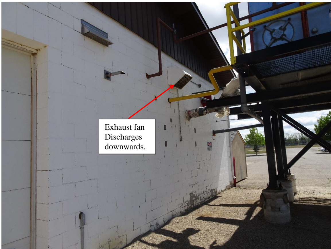
Figure 1 – Fan discharges towards the ground.
