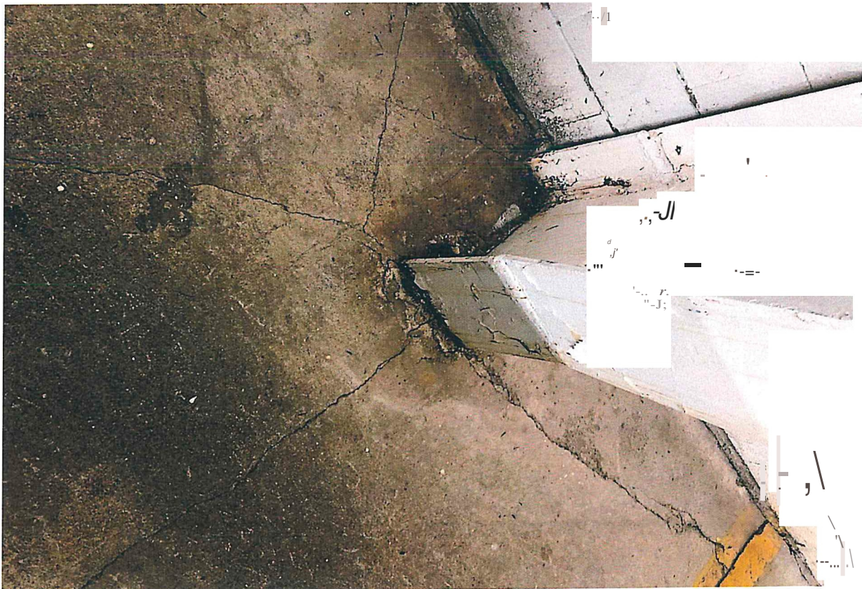
Picture #4 - Substantial cracking at pilaster locations on north side.
