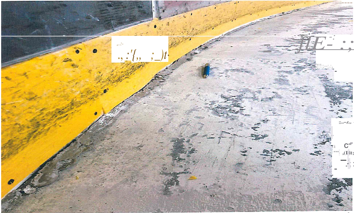
Picture #11 - The gap between the dasher boards and the concrete floor can become pronounced through heaving cycles and caulking requirements become more substantive to prevent water migration beyond the boards. This caulking bead is at least twice the size it should be for water/ice containment.
