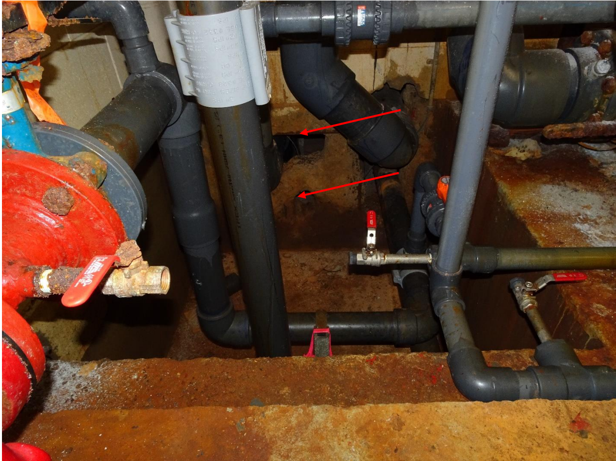
Figure 4 – Brine lines not sealed.
