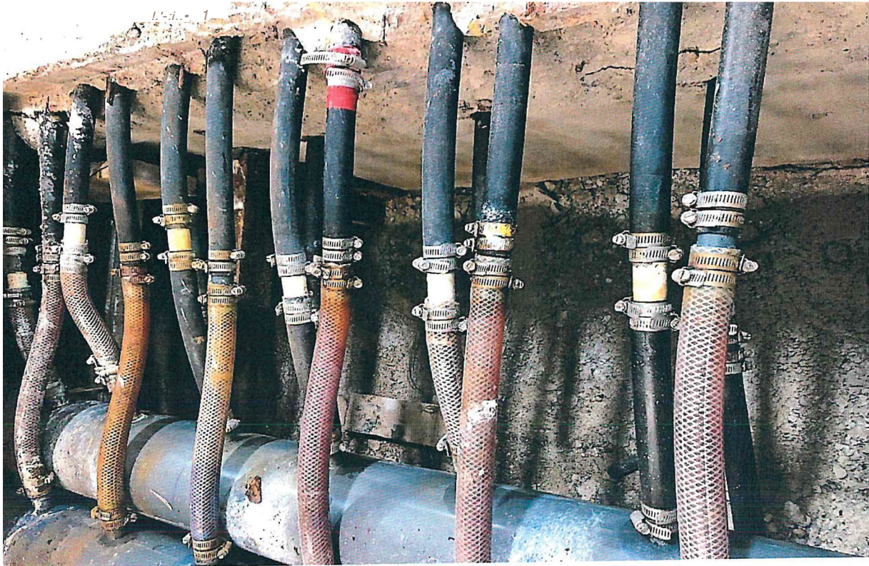
Picture #1 - Spliced rink pipe into 20 year old PVC headers in rough trench
