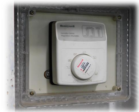
Rink Humidistat Existing Ventilation Control
