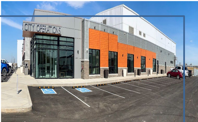
City Operations Centre
