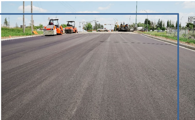
York Road Reconstruction
