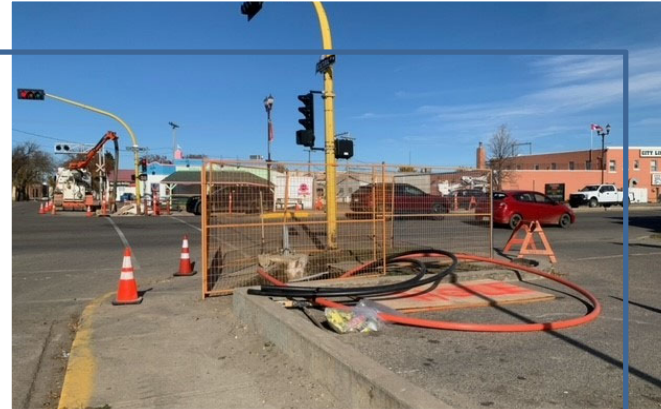
Traffic Signal Pole Replacement
