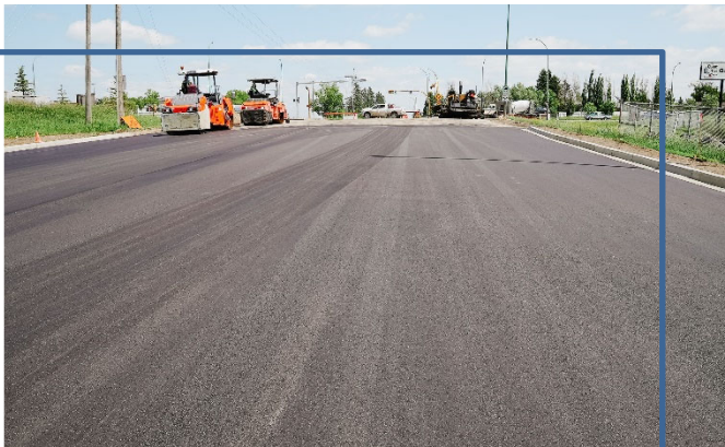
York Road Reconstruction
